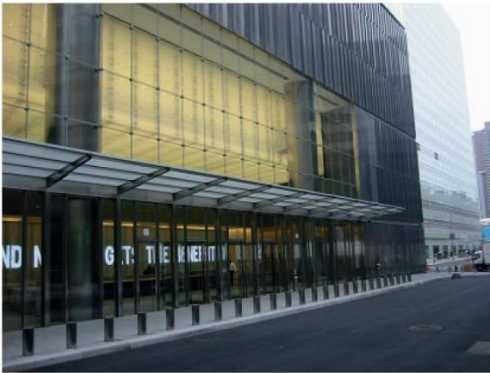
© F. Wellershoff: „Blast enhanced facades for the new World Trade Center Towers“; 2008
